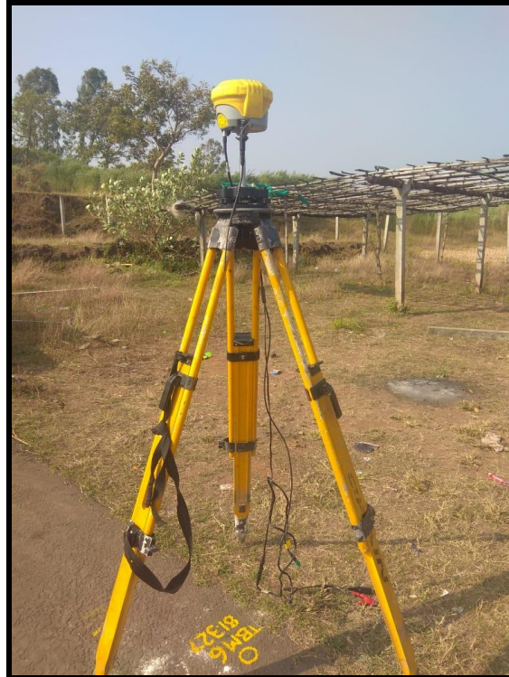
BASE SETUP AT TBM 6
